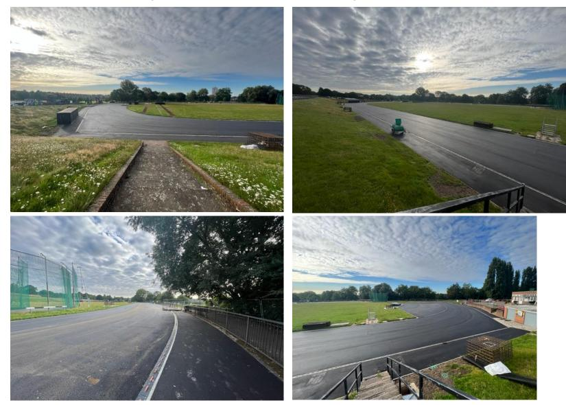
23/08/23 – Track defects made good, additional reconstruction complete using lean concrete mix / mesh in areas.
